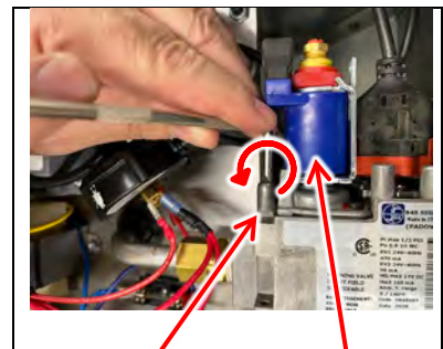
MANIFOLD PRESSURE TAP
